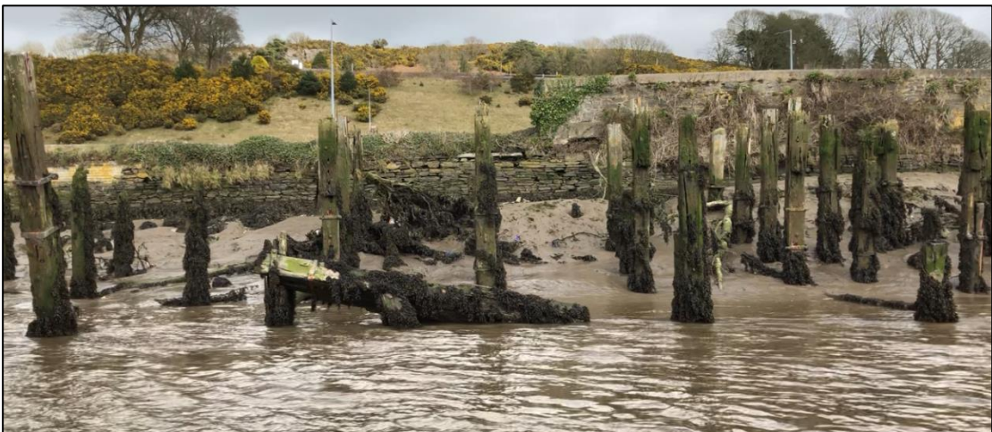
Plate 14.22 Western section of landing stage 7, facing north-northeast
