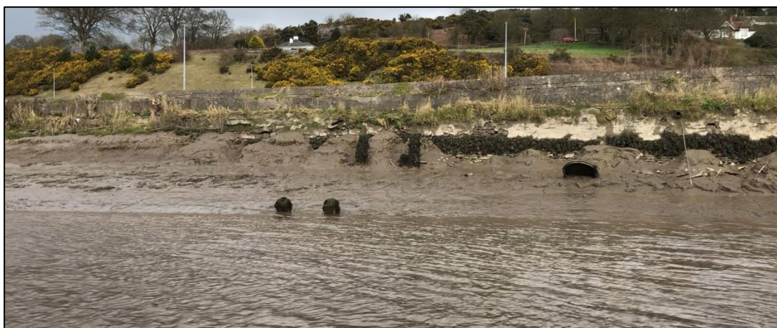
Plate 14.23 Landing stage 8, facing north-northeast
