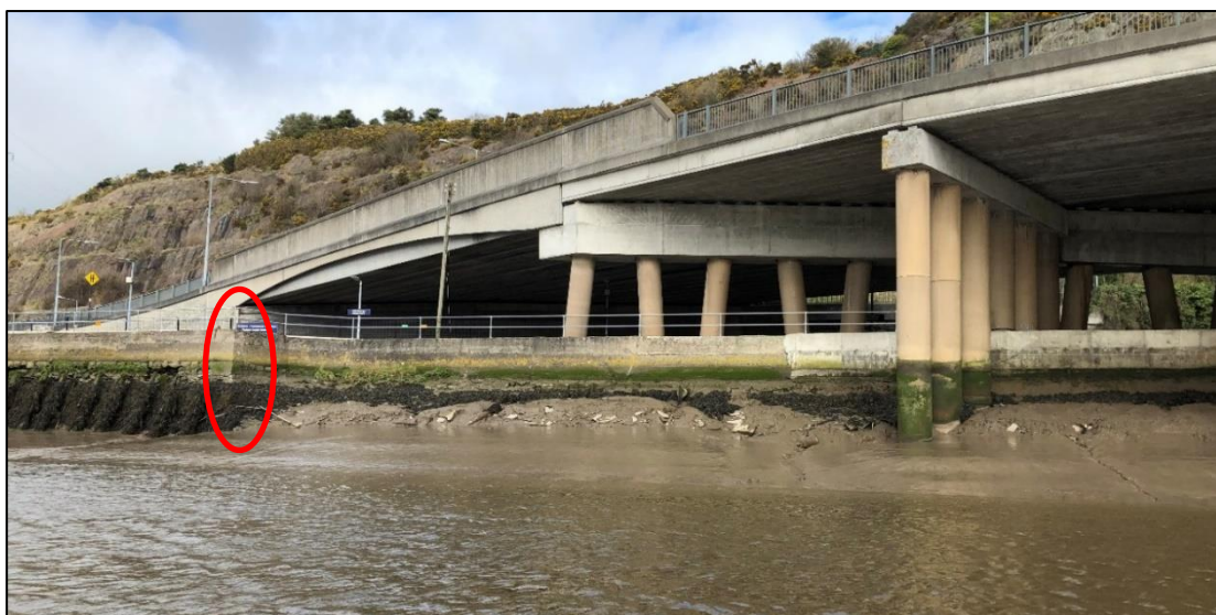
Plate 14.9 Quay wall beneath the R448, facing north
