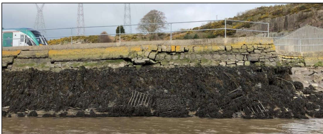
Plate 14.13 Eastern section of landing stage, facing north
