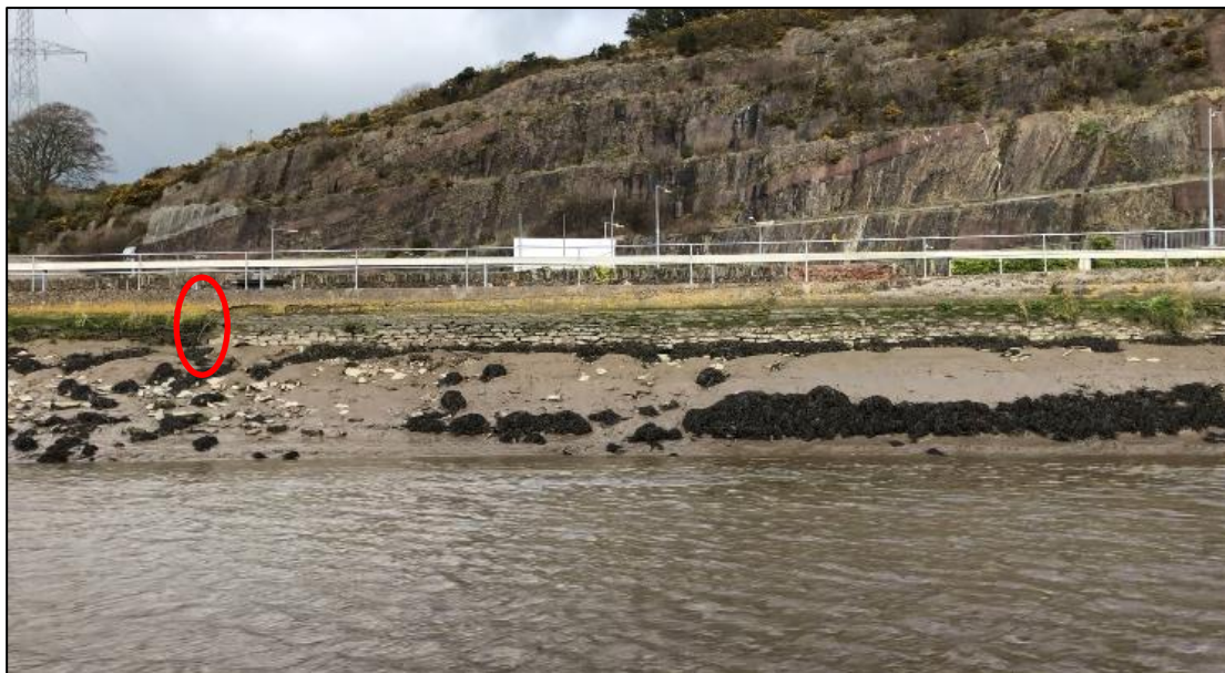
Plate 14.10 Quay wall to the west of the R448, facing north
