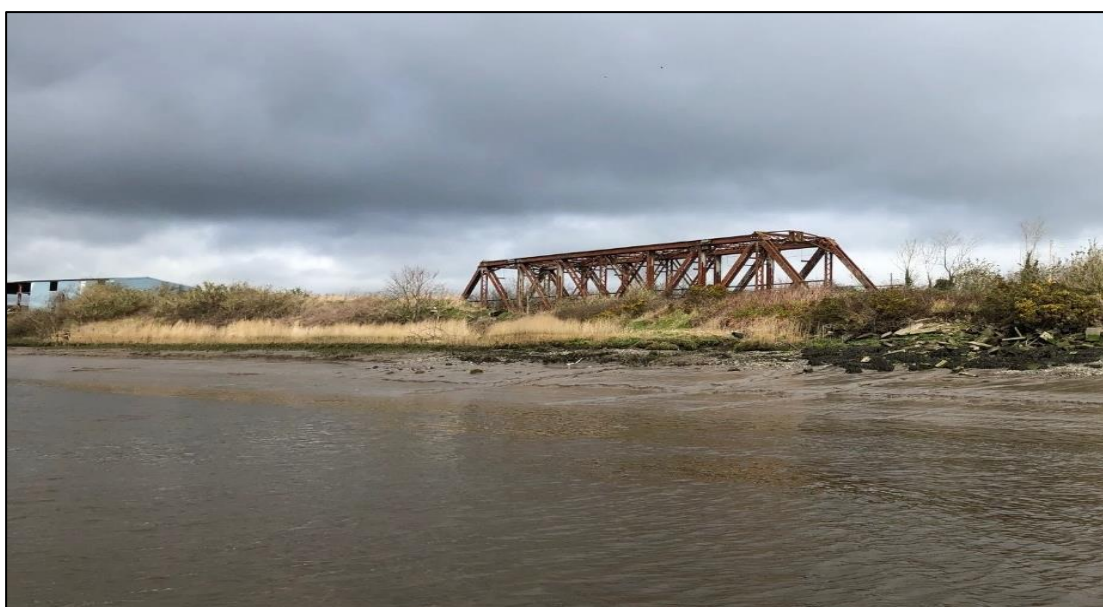
Plate 14.24 Section of iron railway bridge within the compound area, facing north
