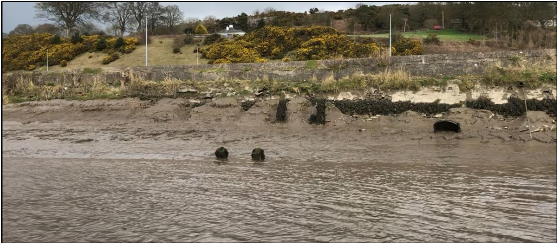
Plate 14.20 Landing stage 6, facing north-northeast
